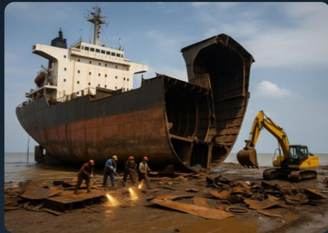
SHIP RECYCLING (HKC compliant Indian recycling yard)
