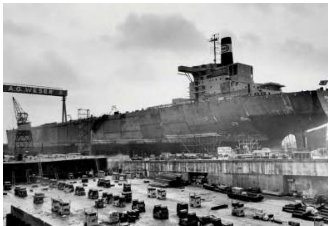
The “Esso Scotia” under construction in the A.G. Weser shipyards in Bremen. The photo was taken on 1 April 1969, a few weeks before the ship’s launch on 31 March 1969. The vessel was built for Esso London, and its capacity of 255,000 dwt made it the biggest tanker built at a European shipyard at the time.
