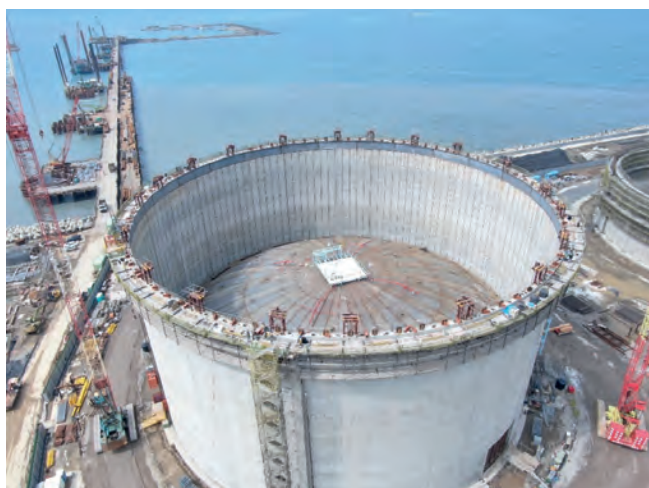
Figure 2. Tank roof air raising for the first tank.
