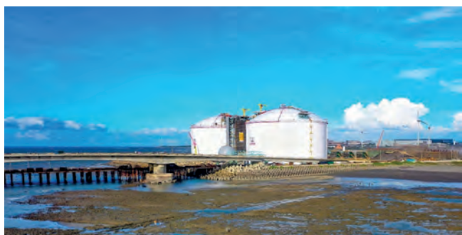
Figure 1. Guantang project is located near the algae reef ecological conservation area. Ecological protection measures must be implemented during construction.
