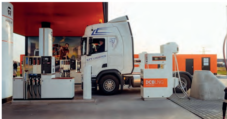
Figure 3. The Netherlands, LIQAL LNG dispenser.
