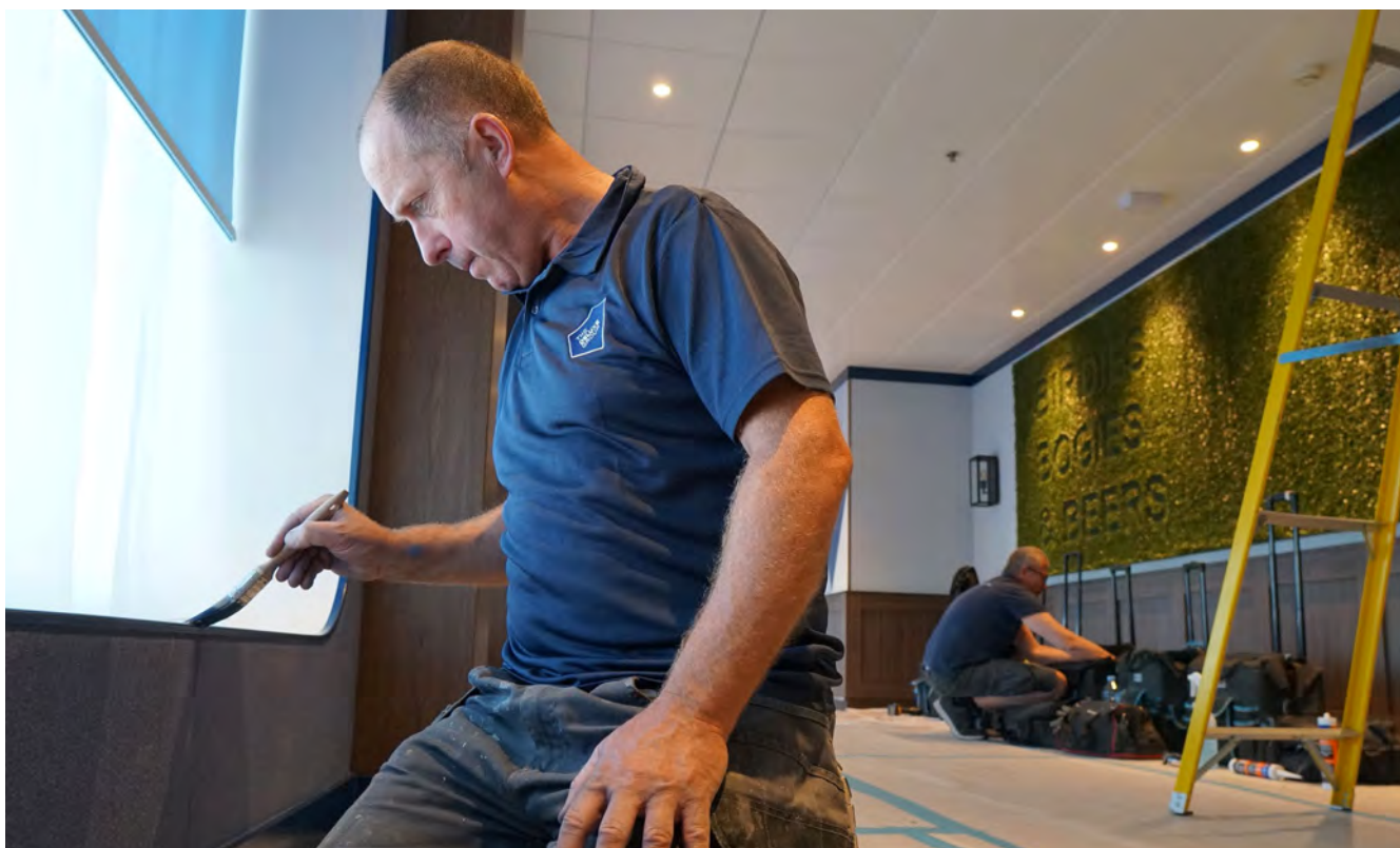
Outfitting firms, such as The Deluxe Group, are experiencing an increase in refurbishment projects onboard older cruise ships
