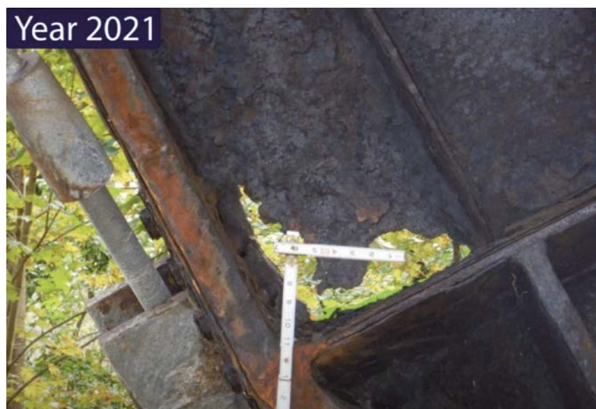
Leg corrosion documented by inspector in 2015, 2017 and 2021 – the year before collapse.
